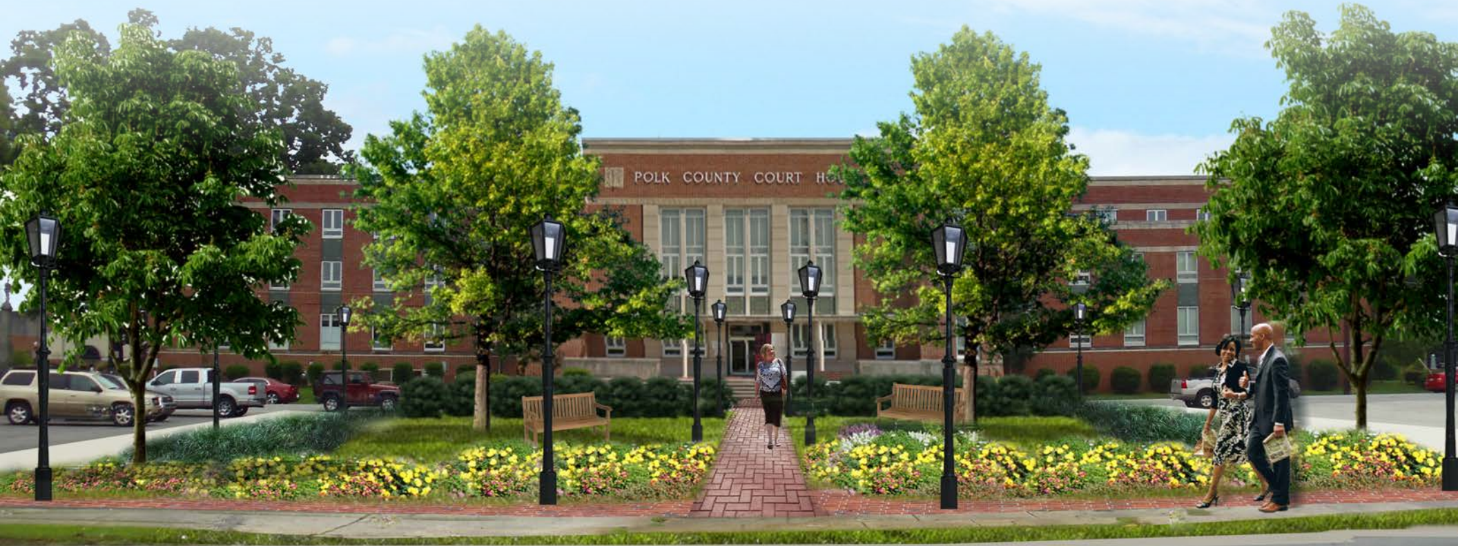
After: This digital rendering shows the Polk County Probate Court addition, parking lot reconfiguration, and landscaping improvements.
