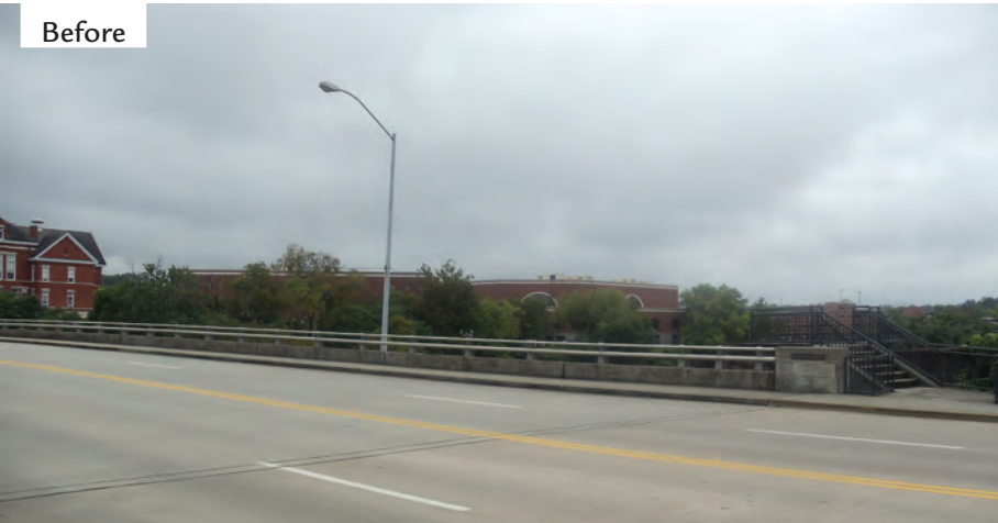
FIGURES 100 & 101. GATEWAY IMPROVEMENTS.
