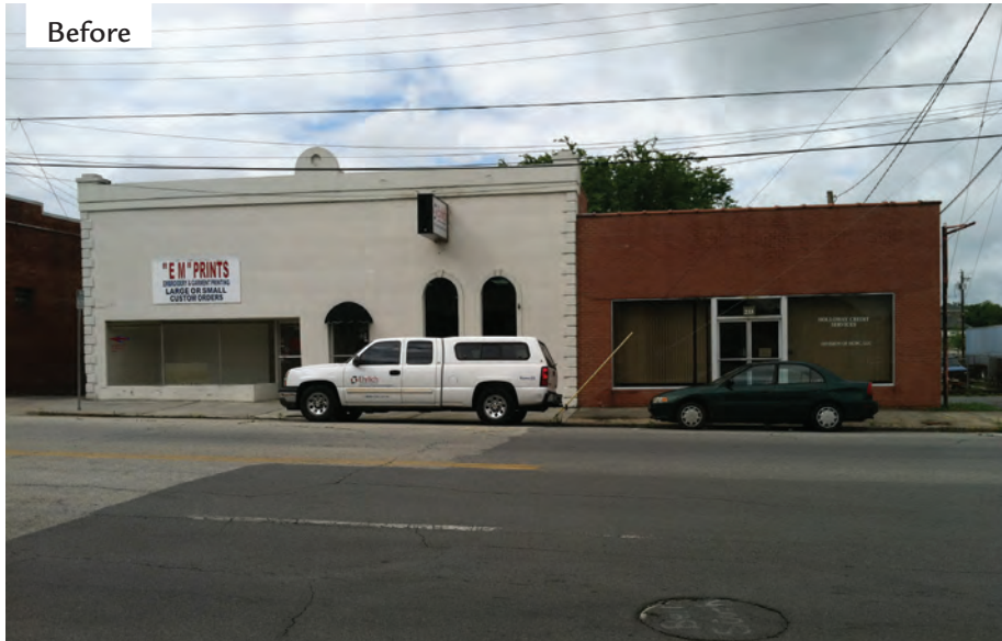
FIGURES 118 & 119. FAÇADE IMPROVEMENTS.
