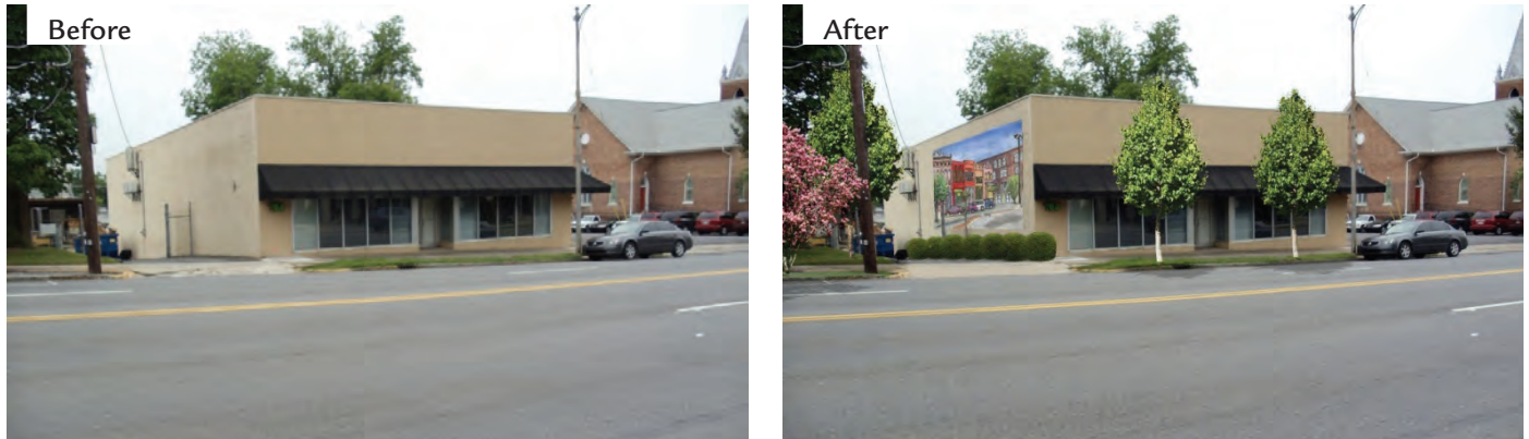
FIGURES 47 & 48, FAÇADE IMPROVEMENTS:
