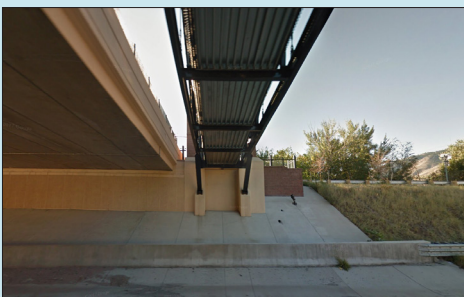
GOLDEN, COLORADO PEDESTRIAN BRIDGE EXAMPLES
